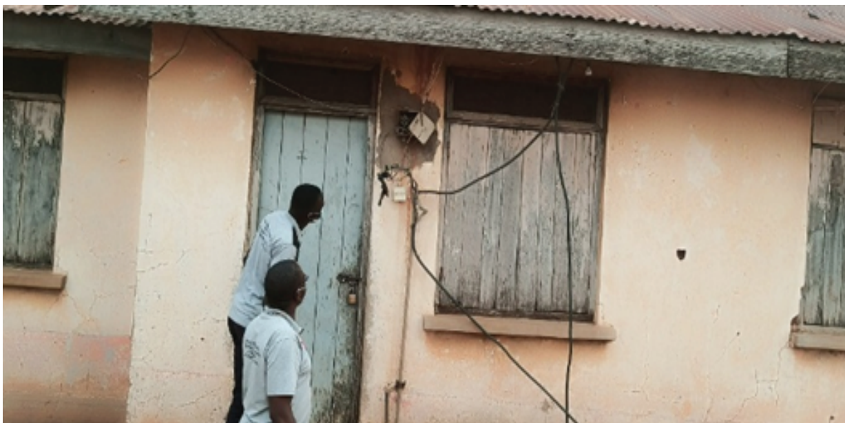
Dangerous connections to electricity at a police barracks in Northern Uganda
