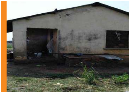
Building occupied by Lamwo CPS in Padibe
