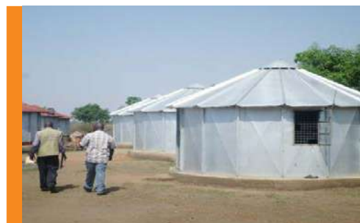
Newly constructed uniports at Ragem Prison in Nebbi district
