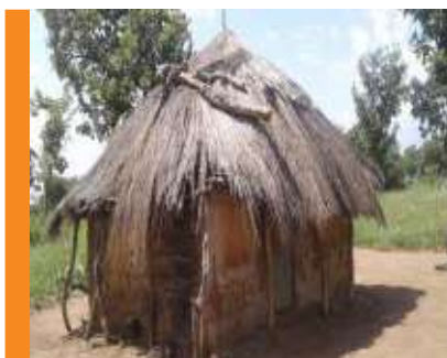
Police accommodation at Ogor Police post, June 2017
