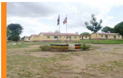
Staff quarters recently renovated at Koboko Prison
