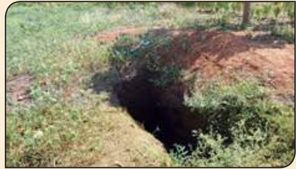
An open pit latrine- A health hazard
