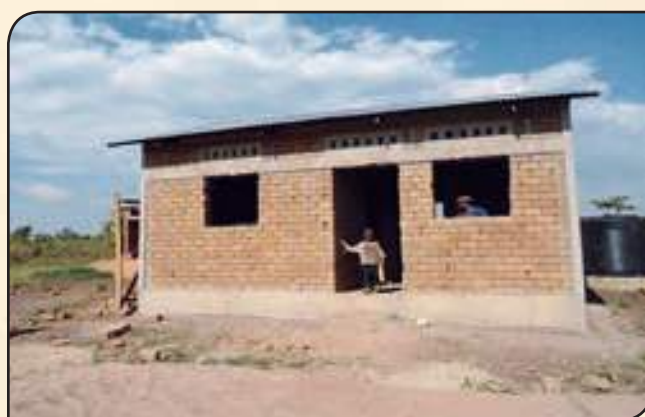
A four roomed house being constructed by Habitat for Humanity
