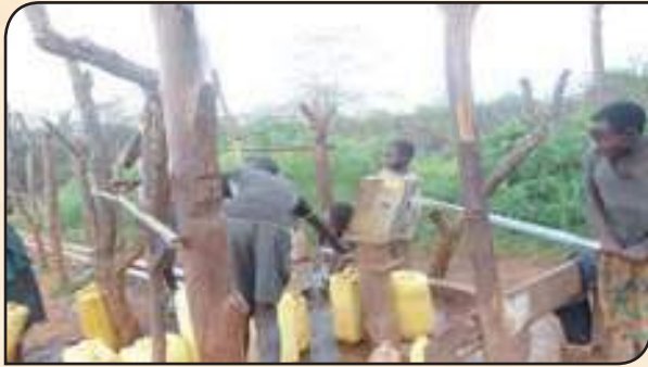
A bore hole in the resettlement camp
