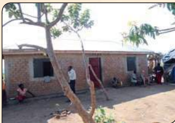
A completed three roomed hydraform house by the Office of the Prime Minister
