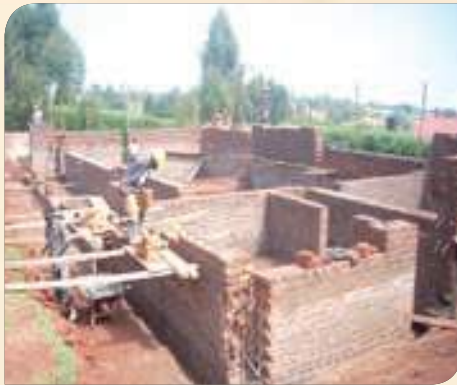
On-going Construction work on 2 new wards for male and female inmates at Kapchorwa
