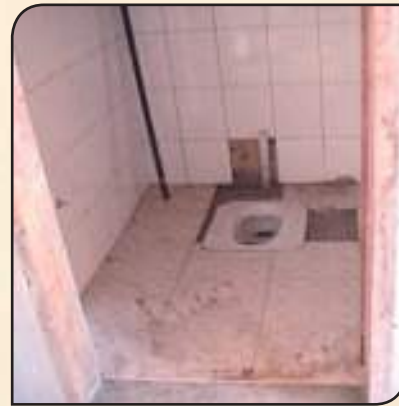
A toilet in one of the wards under renovation at Kibaale Prison
