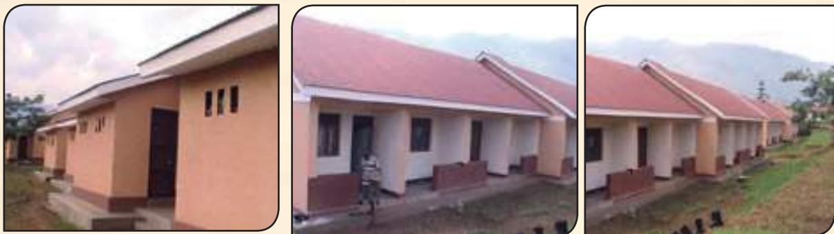
Newly constructed staff buildings at Bundibugyo Police station
