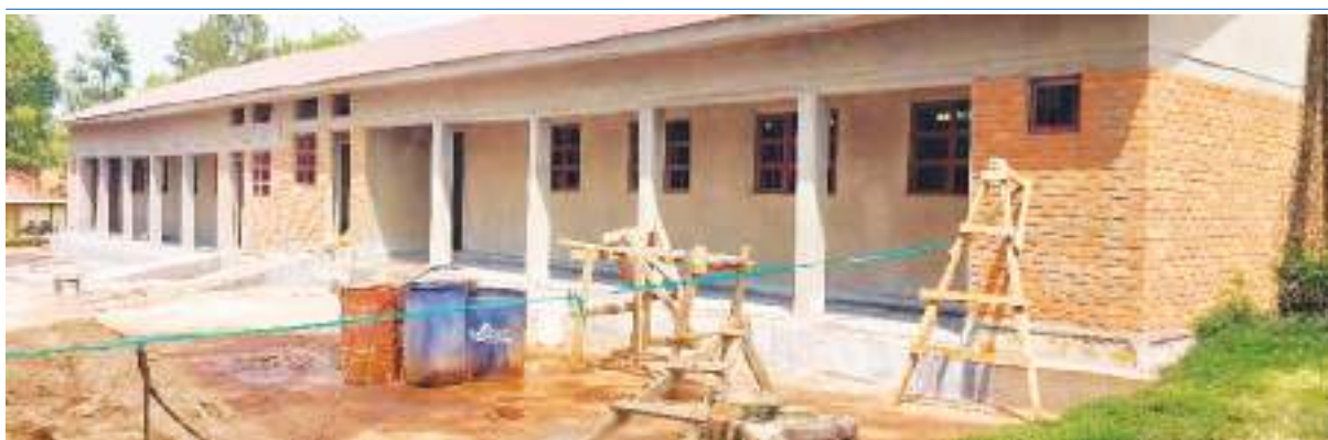
Newly constructed twin male ward at the prison in Isimba in Masindi District. © UHRC
