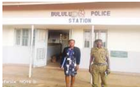
A modern Police station at Bululu Police Station in Kalaki District. © UHRC
