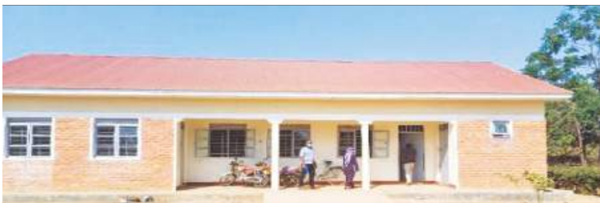
Newly constructed permanent female ward, including a water-borne toilet facility with flowing water at Amolatar Prison. © UHRC
