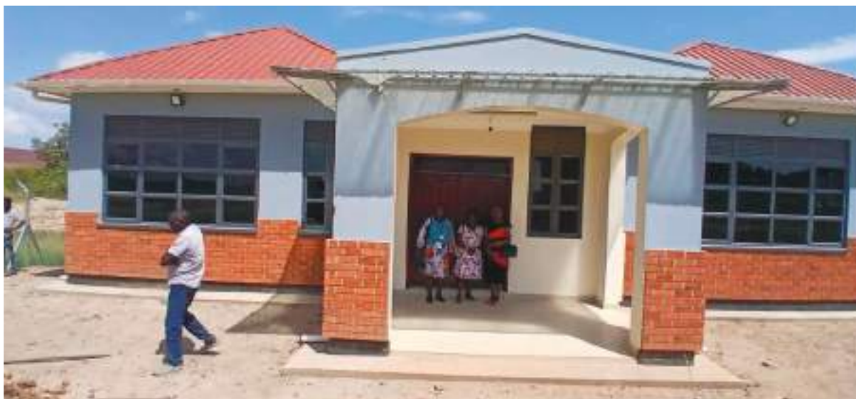
UHRC Moyo Field Office block as at December 2025 © UHRC
