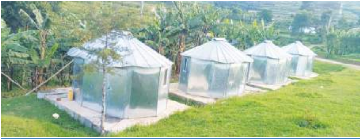
Newly erected uniports at Maziba Police Station. © UHRC
