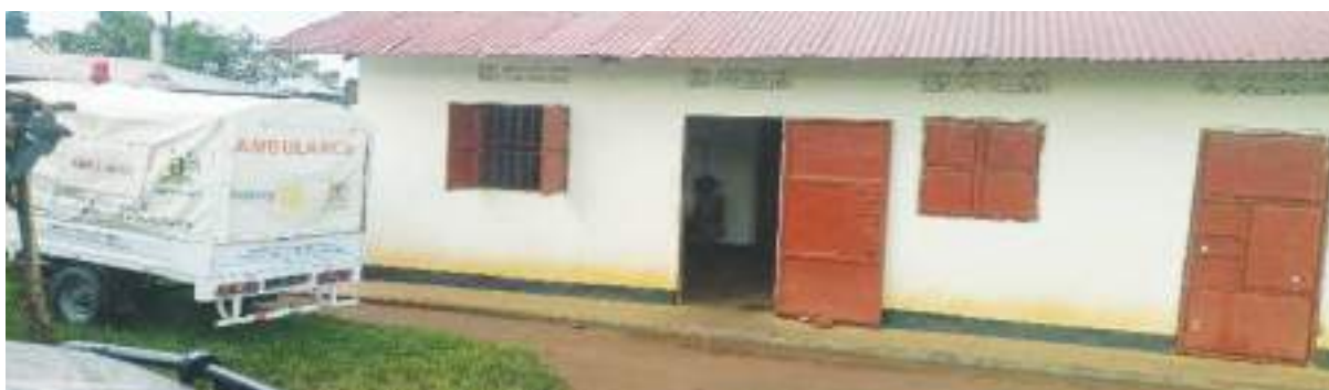
Newly fixed metallic doors and windows at Kateete Police Station. © UHRC
