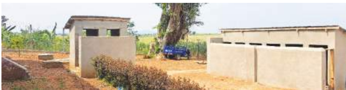
Newly constructed pit latrines at the prison in Maiha, in Masindi District. © UHRC
