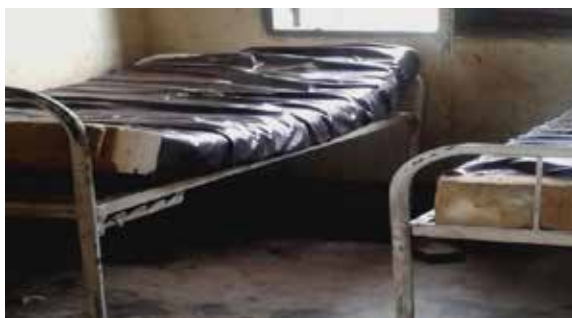
Worn out beds in the antenatal ward at Lwengo HC IV Lwengo District
