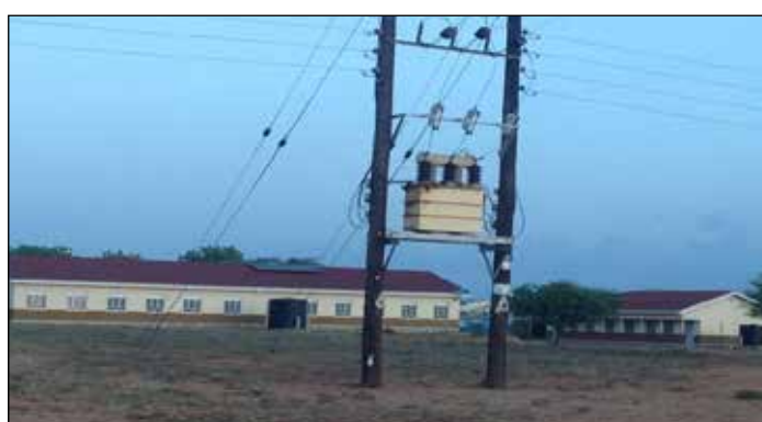
Pokot Secondary School in Amudat District, is one of secondary schools opened during disarmament
