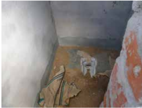
Water borne toilet under construction at Kotido Prison
