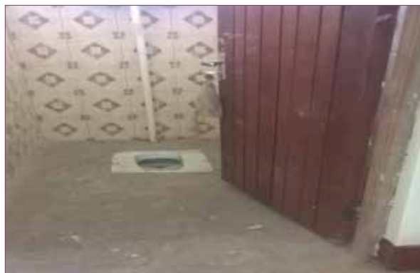
A flush toilet at the newly constructed Mutukula Prison Farm complex
