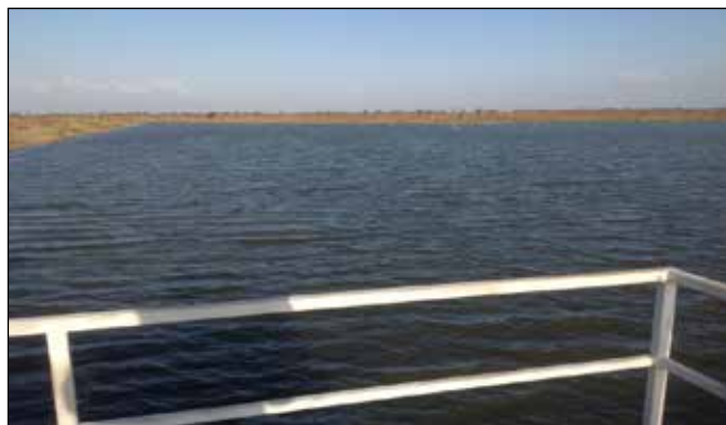
Arecek Dam in Napak District
